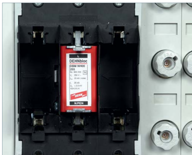
DBM NH00 255: Coordinated single-pole lightning current arrester in NH00 design with high follow current limitation for U c = 255 V
