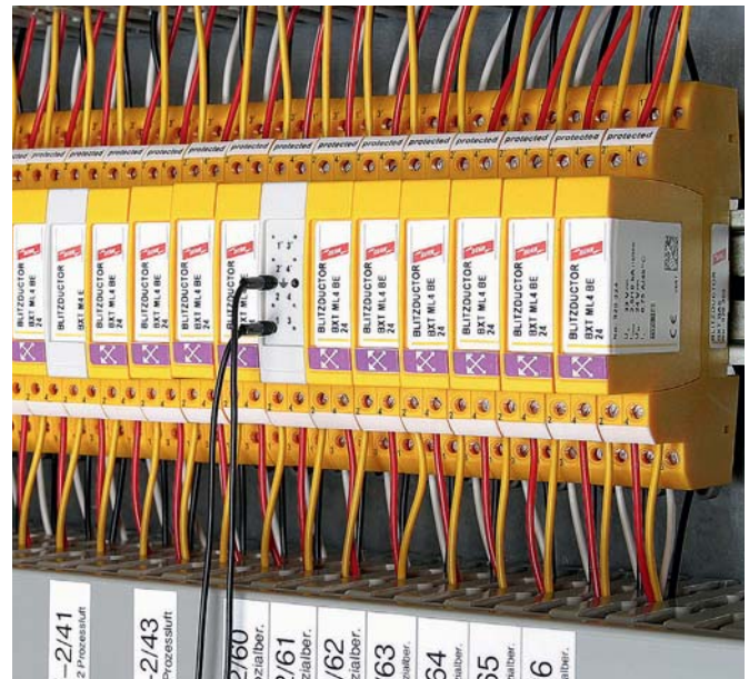
BLITZDUCTOR XT with an earthing module (grey). The lines can be tested by means of the measuring module (grey with lines) without disconnecting the terminals.
