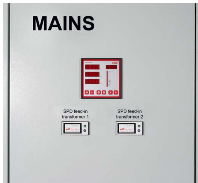
Visual indicator for surge protective devices for installation into switchgear cabinets.
