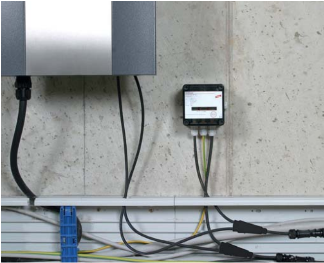
Prewired connecting cables for easily connecting the incoming string lines to DEHNcube and the inverter.
