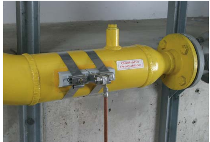
Pipe clamp for electrical contacting of pipes in explosion-hazardous areas for implementing of lightning equipotential bonding according to IEC/EN 62305-3
